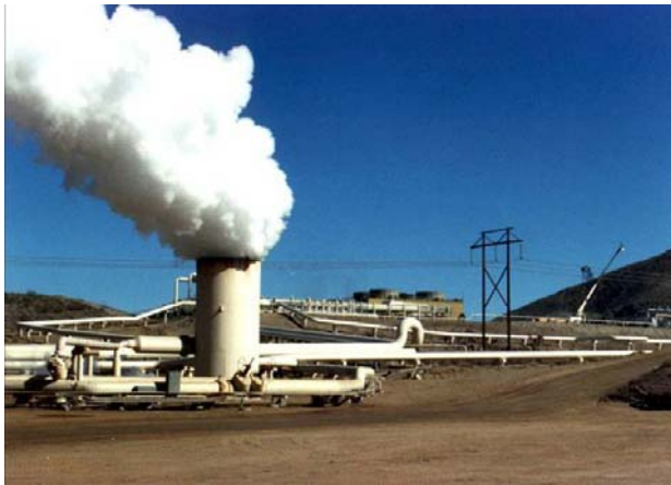
Figure 25: Flowing Steam Through a Silencer at Coso, a Double Flash Plant in California
