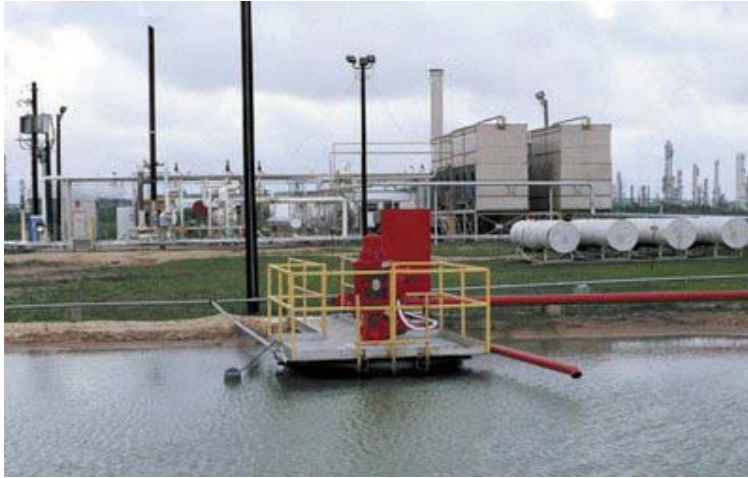
Figure 16: Geopressed Demonstration Plant in Texas
