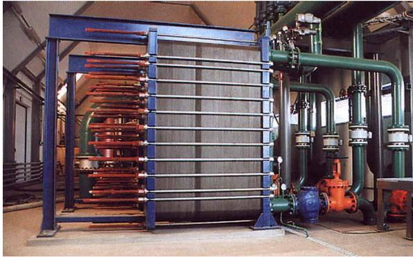
FIGURE 4.10: Geothermal base load plant, Banska Nizna – plate heat exchangers (photo T. Kliszczy)
