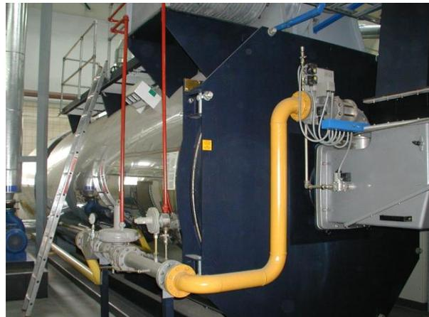
FIGURE 4.12: Central peak load plant, Zakopane – inside view (photo T. Kliszczy)
