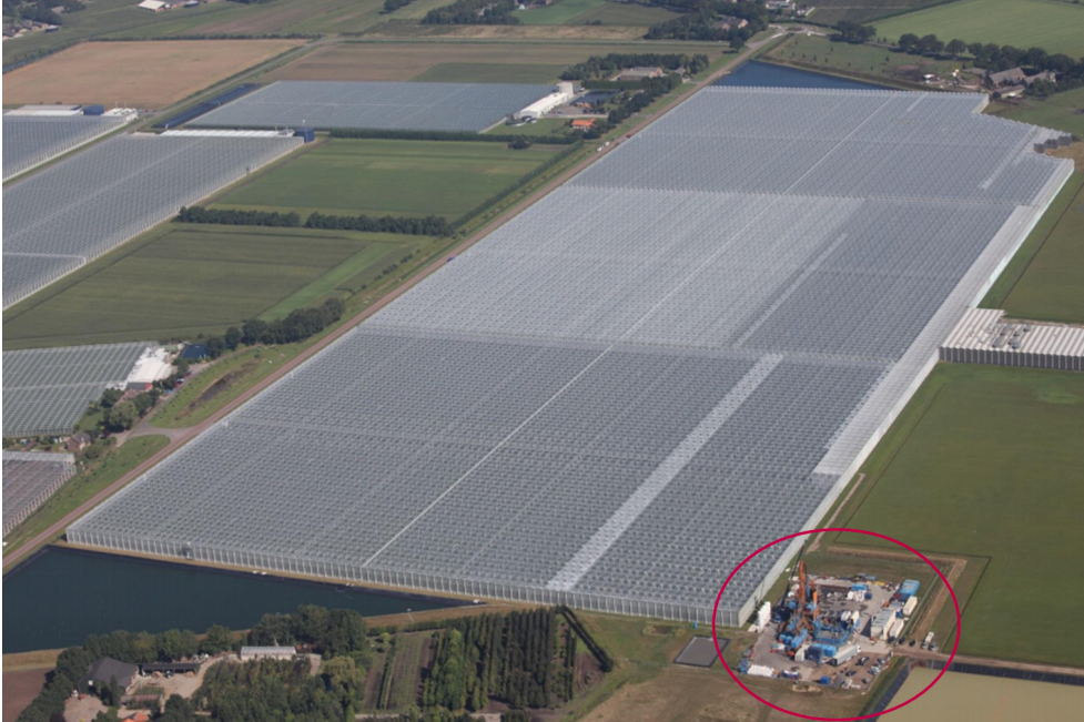
Fig. 2.1. This aerial photograph of the construction site and greenhouses at Van Wijnen Square Crops in Californië, Limburg. Source: [96]
