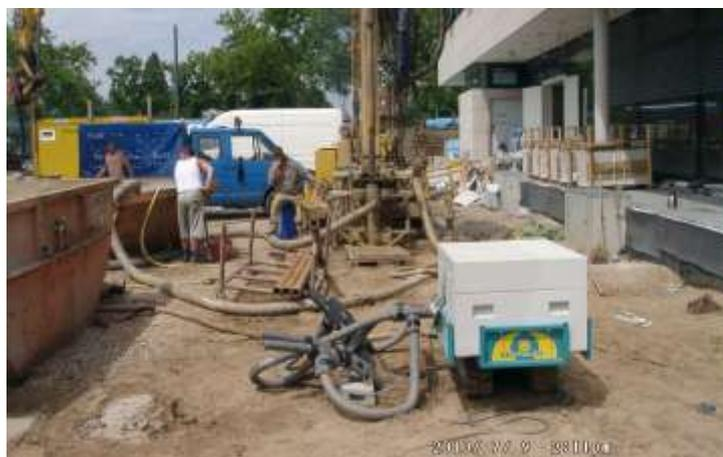
Figure 6: Make sure that there is no drilling work near the test-BHE. Preferably there is no drilling during the test at all. The drilling in near surroundings may induce a groundwater flow that disturbs the TRT
