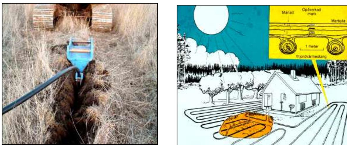
Fig.3. The horizontal loop system that requires large open space to be applied
