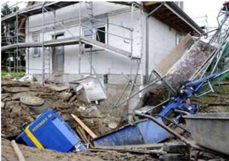
*Figure 2. An undermined ground collapsed and caused damages*
