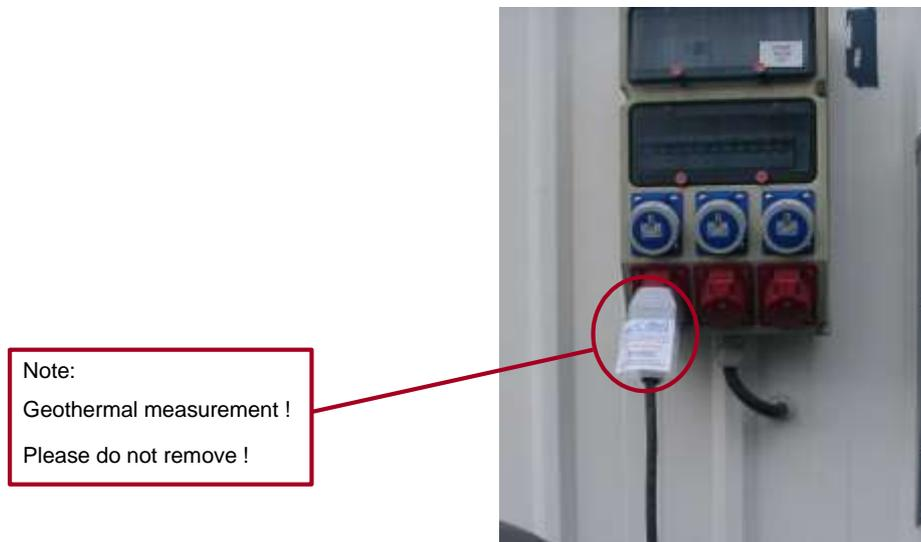
Figure 8: Make sure that no one interrupts your power supply. Sometimes simple things are of great value!
