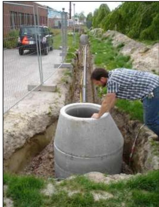
*Fig 4. Drillers are occasionally responsible for delivering the well houses. Here examples of house placed on the ground and one simpler dug down beneath the surface.*
