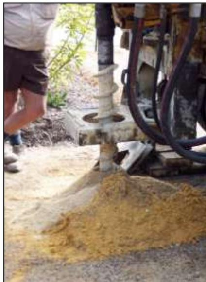
Figure 5. Auger drilling that in this case is done with hollow stem equipment.
