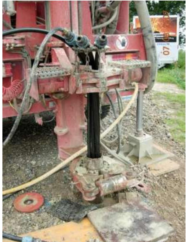
Figure 7. During grouting the auxiliary casing still prevents the borehole from collapsing. The BHE is under pressure (picture: Polydynamics Engineering Zurich)
