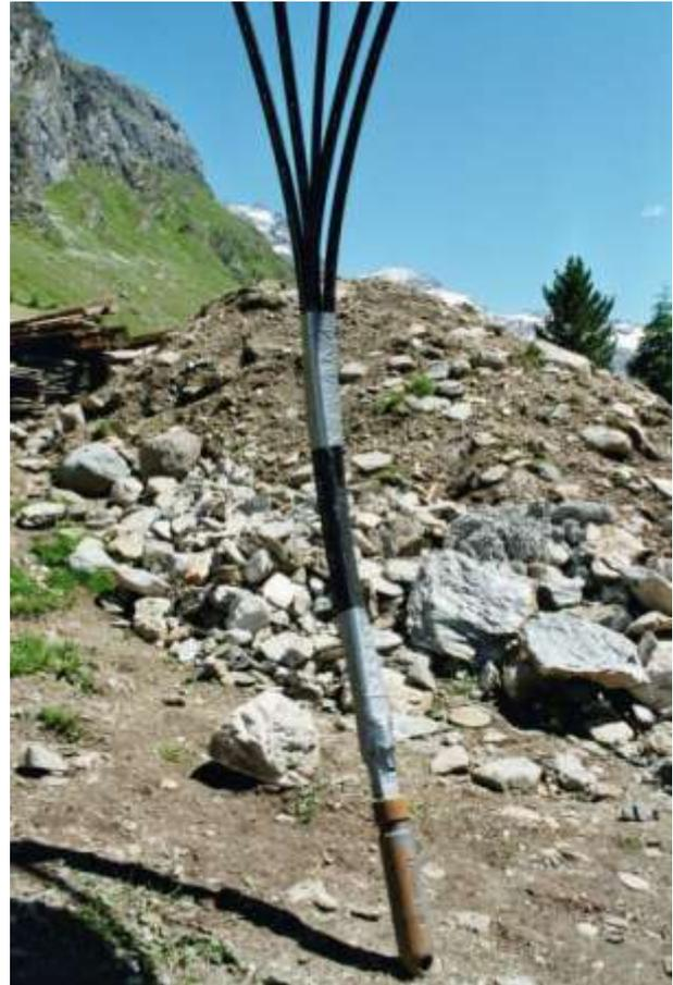
Figure 2. Ready-to-insert BHE with an additional weight, protected foot and a fifth injection tube
