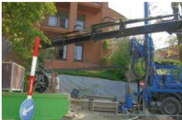
Figure 4. Guide rollers to ensure vertical insertion (picture: Polydynamics Engineering Zurich)
