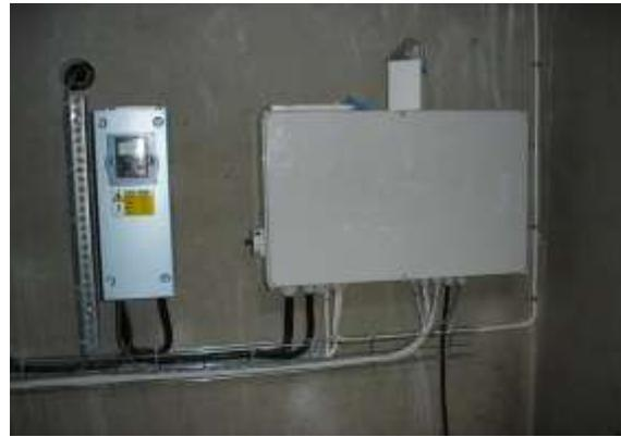
*Fig.1 Submersible pump with motor and impeller and the intake of water placed between. The next image shows a box for frequency control (left) and a box for electrical connections for the pump and controlling devices in and close to the well (right).*
