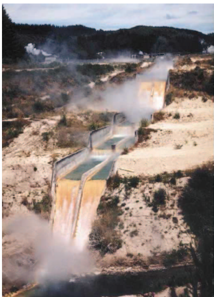
Fig.4.3.1. Geothermal fluid drain at Wairakei, New Zealand geothermal site. Silica precipitate of orange-brown color line the channel
