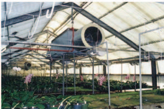
Fig.7.49. Horizontal air heating units
