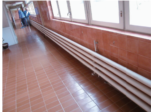
Fig.7.27. Simple steel pipe heating system
