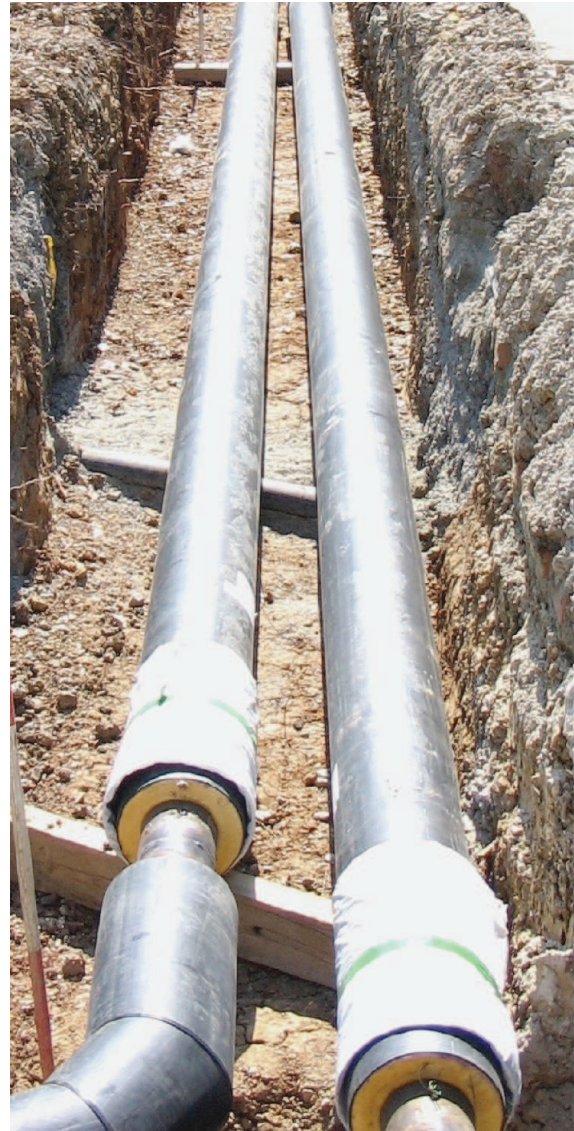
Fig.7.9. Buried pipes installation
