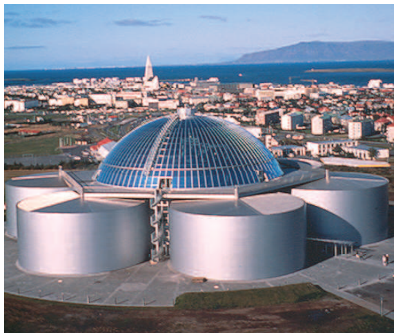
Fig.7.22. Heat accumulators of the Reykjavik (Iceland) district heating system
