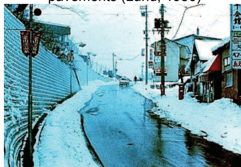
Fig.7.70. A street in Japan with snow melting installation
