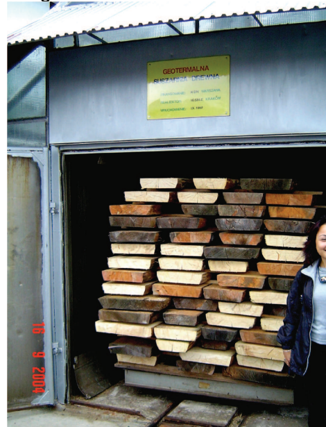
Fig.7.61. Timber drying chamber (Zakopane, Poland)
