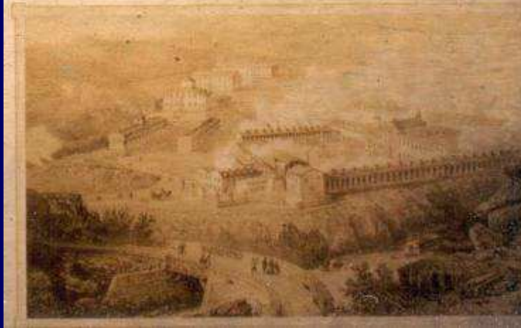
The "Factory" in Larderello, 1850. Natural thermal energy was used to extract boric acid from nearby pools. Later the geothermal steam was used to produce electricity.
