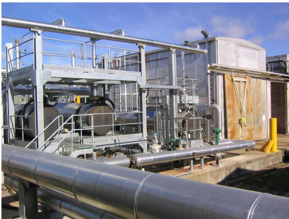
Figure 4.7. Recently commissioned Contact Energy geothermal heat supply to the Tenon kilns at Taupo (courtesy of Contact Energy).
