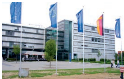
Office building in Germany, baseload heat and cold provided by heat pump connected to 154 BHE
