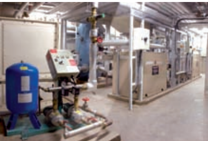
Geothermal groundwater heat pump for Glucksman gallery, Cork University, Ireland
