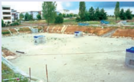
The BTES in Neckarsulm under construction (>500 BHE)
