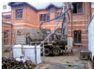
Renewable Energy House in Brussels, Belgium, drilling for 4 BHE and schematic
