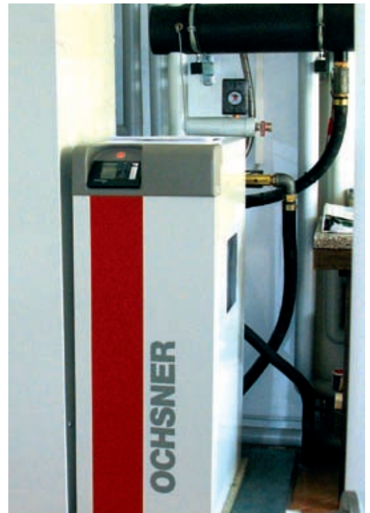
Small residential house in Germany, using direct expansion horizontal collector and small heat pump
