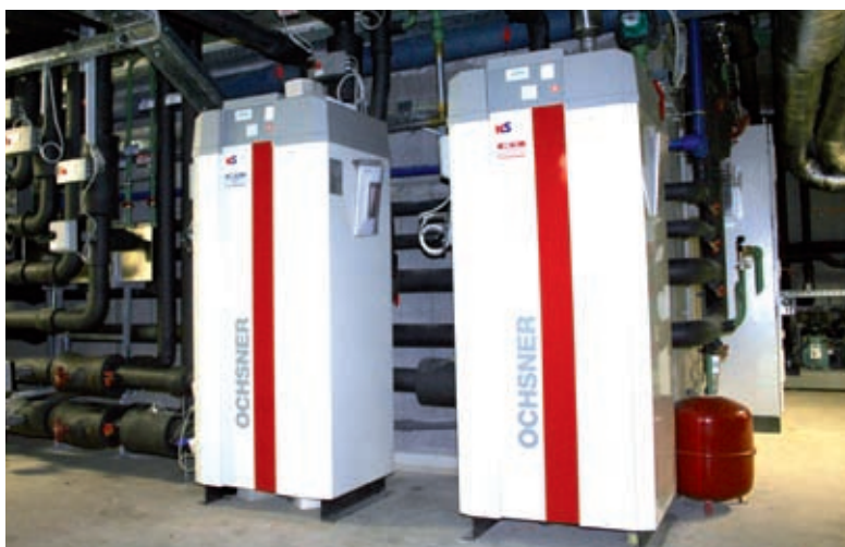
Supermarket for eco-food in Austria, heated and cooled by heat pumps on groundwater wells
