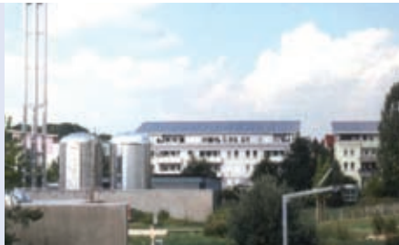
Houses with solar collectors in Neckarsulm, Germany
