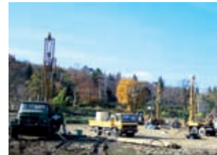
BHE drilling and manifold installation for office building in Törökbalint, Hungary
