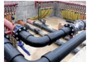
BHE drilling and manifold installation for office building in Törökbalint, Hungary
