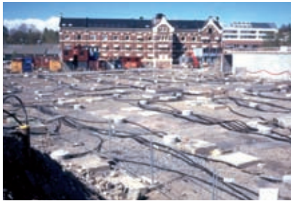
Geothermal groundwater heat pump for Glucksman gallery, Cork University, Ireland
