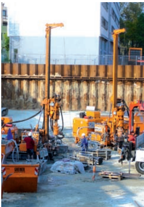
A drilling site
