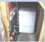
Fig 1: Picture features 8kW heat pump unit connected to the ground loops via the red manifolds. Picture courtesy of Kensa Engineering.
