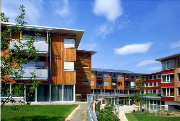
Figure: Building just finished
