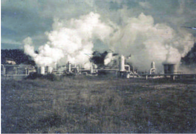
Figure 9. Wairakei, New Zealand geothermal field.
