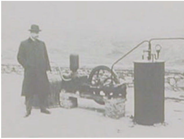
Figure 3. Prince Ginori Conti and the 10-kW experimental power plant, Larderello, Italy, 1914 (courtesy of ENEL).
