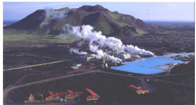
Figure 16. Combined heat and power plant at Svartsengi, Iceland—Blue Lagoon on right (courtesy of Haukur Snorrason, Reykjavik, Iceland).
