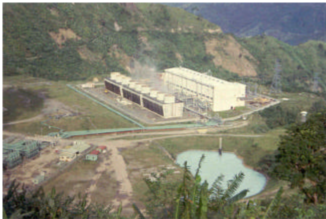
Figure 12. Modern 110-MW plant at The Geysers, California.
