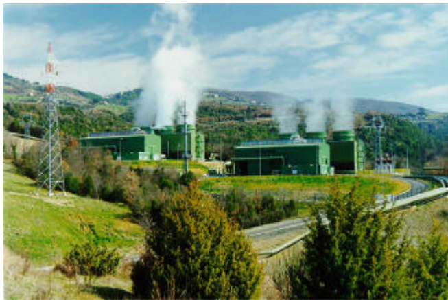
Figure 7. Geothermal power plant at Larderello today (courtesy of ENEL).
