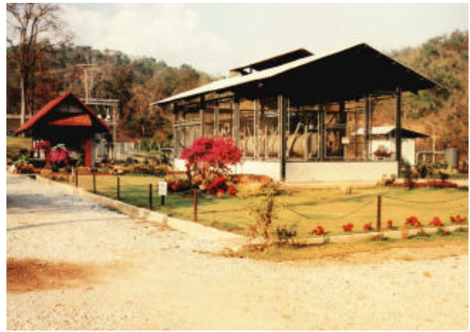
Figure 18. Binary power plant, 300 kW, at Fang, Thailand (courtesy of ORMAT).
