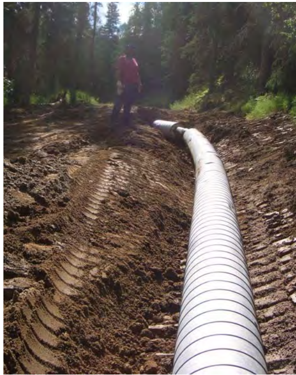
Figure 17. Installation of Hot Water Supply Pipeline
