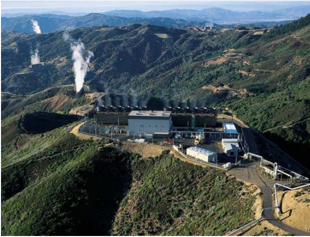
Figure 7: The Geysers, CA, Dry Steam Plant
