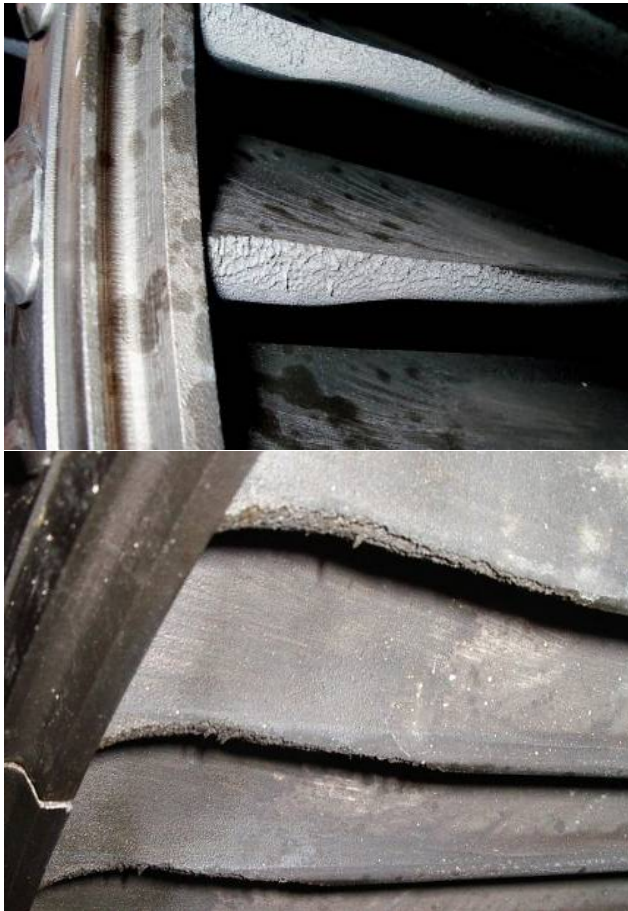
Figure 10. Erosion of turbine mobile and fixed blades.
