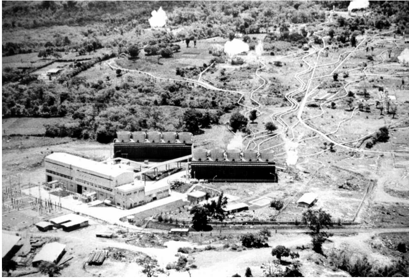
Figure 8.2 Ahuachapan geothermal facility after commissioning around 1977 (DiPippo, 1978).
