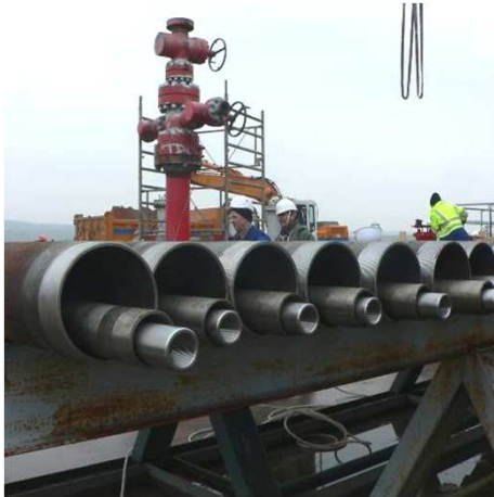
riser, enclosing tube, shaft
